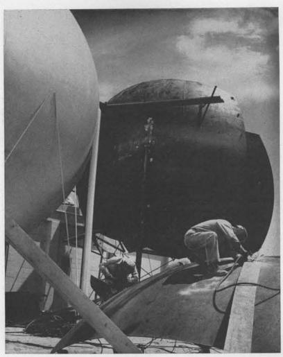
NEW WIND TUNNEL TANK takes form as welders assemble sections of the sphere. A second new tank will also be installed and both should be completed by mid-August. Contractor for the project is Lluts Construction Co. Pittsburgh-Des Moines Steel Co. is installing the 10,000 cu. ft. vacuum tanks. They will be utilized as part of Sandia's new hypersonic wind tunnel facility now being built in Bldg. 865. Randy Holt (4543) is project engineer.
